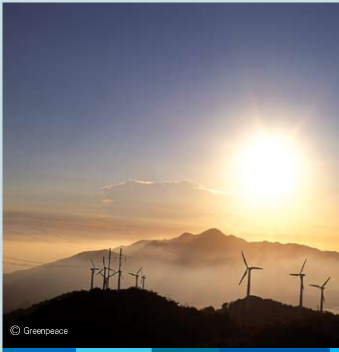
广东南澳风电场 Wind park in Nan'ao, Guangdong
